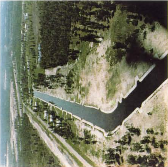
AERIAL VIEW OF AN IP CANAL Sloping clean neat concrete walls with boat slip at each homesite.
